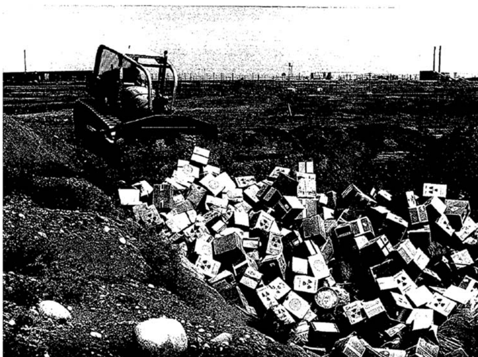
Figure G.2-7. Covering boxes with radioactive contents disposed 618-11 trenches with soil, from HNF-EP-0649 Rev. 0, 1997.
