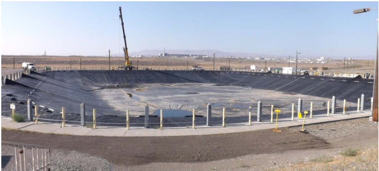
Figure H.12-5. LERF Floating Cover Support System 31
