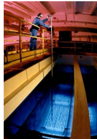
Figure ES-1-10. DOE photo of cesium and strontium capsules in the WESF pools.
