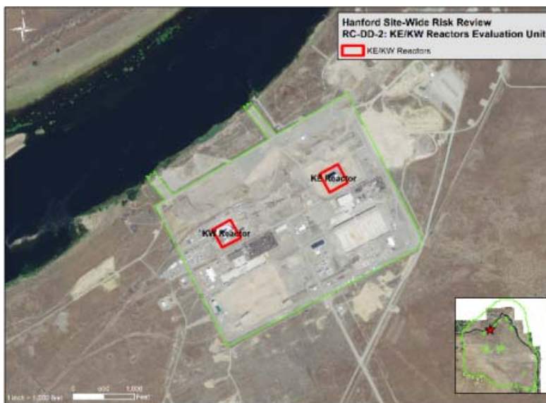
Figure 3-48. Aerial view of K-East, K-West reactors
