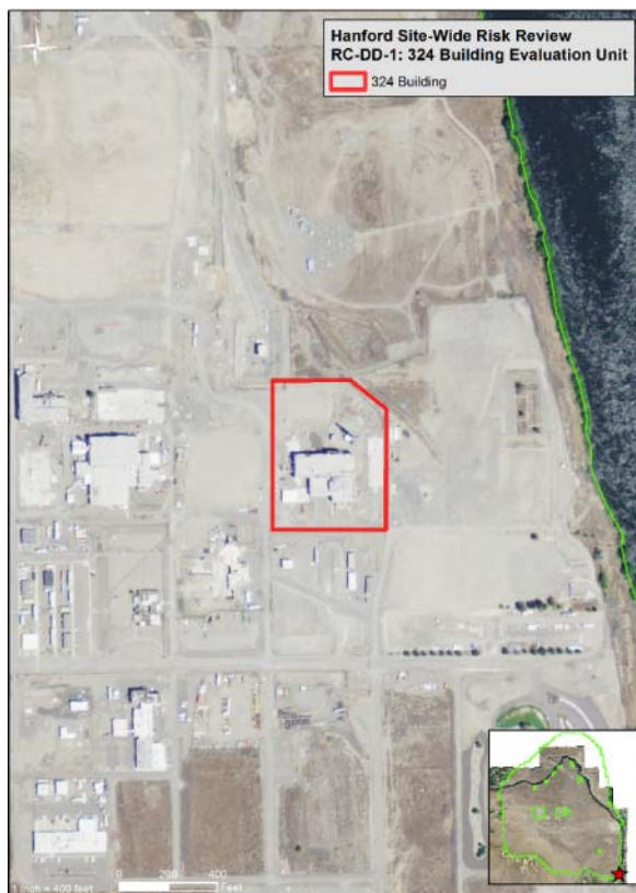
Figure 3-47. Aerial view of Building 324.
