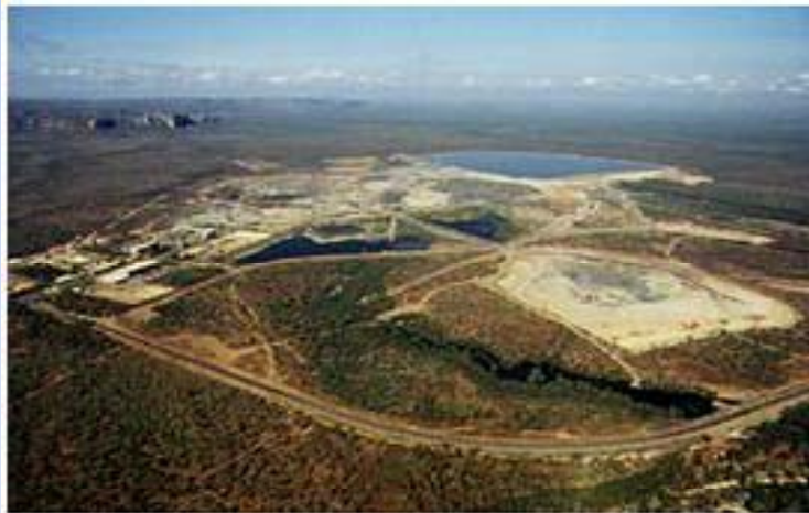
Aerial view of Ranger Mine and plant
