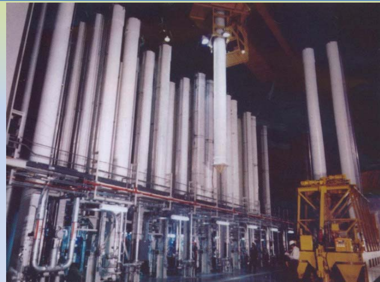
Installation of centrifuges in USEC Plant
