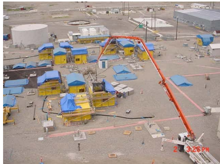
Tanks being Grouted
