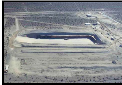
LLW Disposal Engineered Trench
