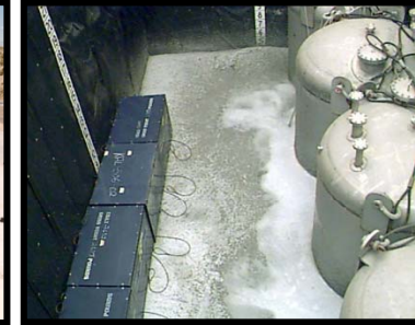
LLW Disposal Grouted in Vault
