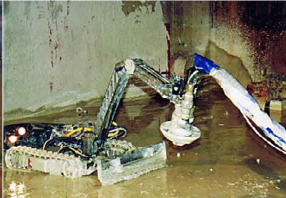
Retrieval of tank waste
