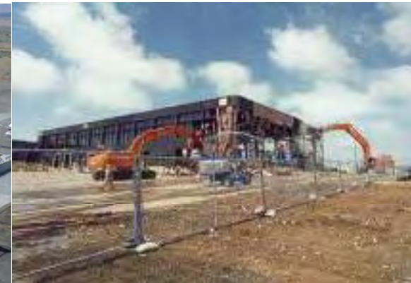
Decontamination and decommissioning (D&D) of hundreds of facilities
