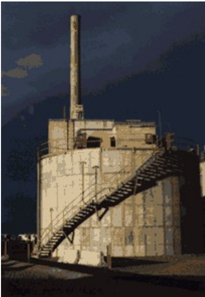
Figure 2. Photograph showing the above ground portion of a bin set.
